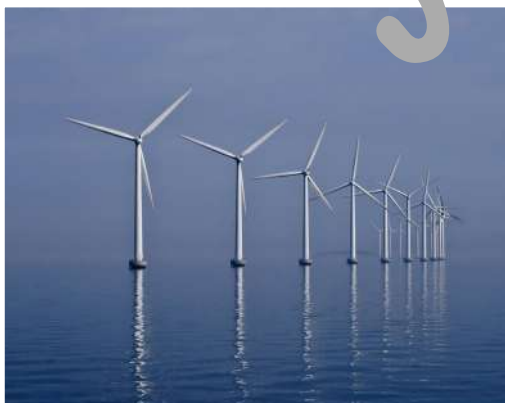
Figure 9: Windfarm in the sea
