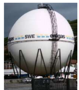
Figure 3: Storage tank for natural gas above ground
