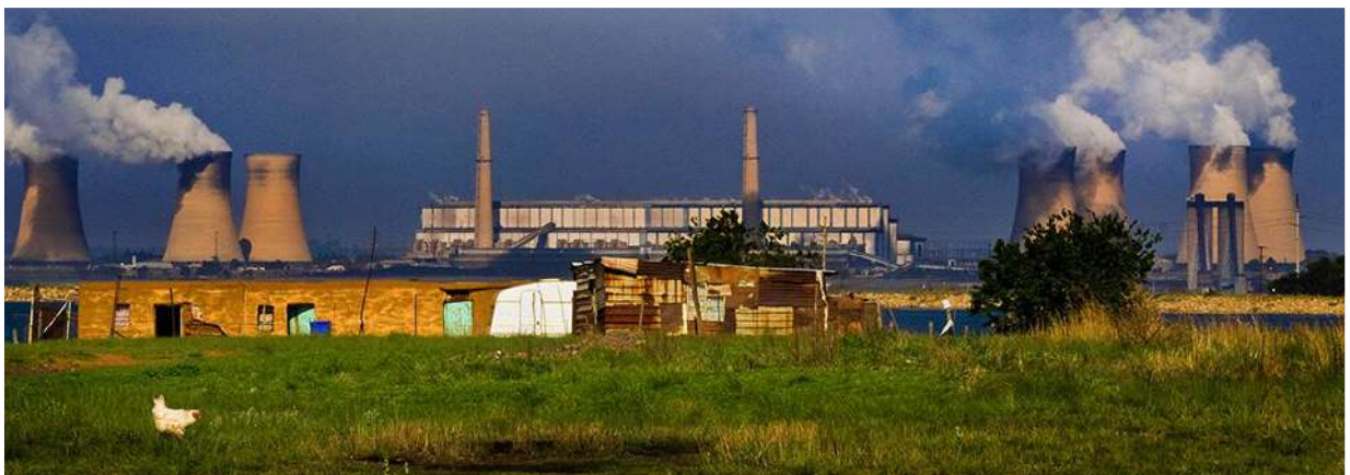
Figure 10: Hendrina coal power station.
